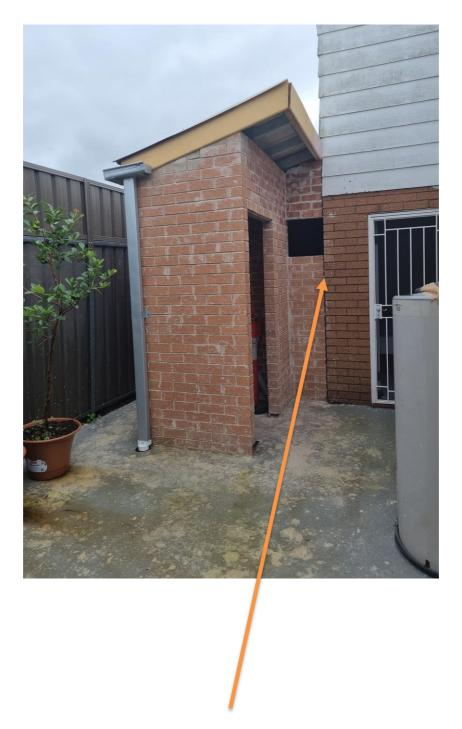
There is no bracing for the new brick work to the existing brick walls
