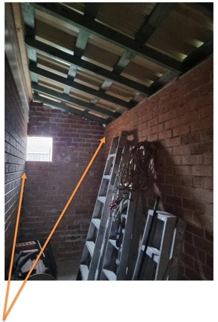
Engaged pier are missing to tie up the corner
