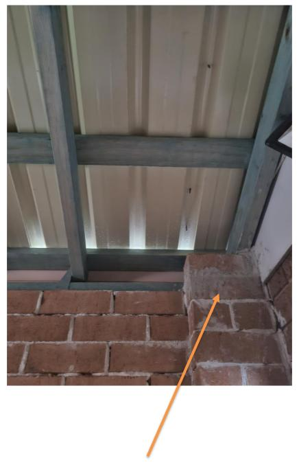
Missing Strap from brick pier to top plate as per AS1170
