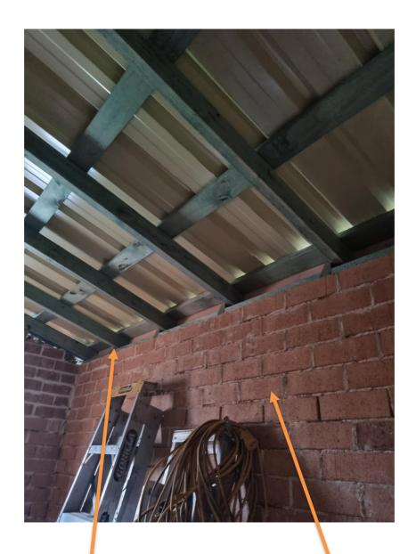
Strap for up lift wind pressure on each rafter
